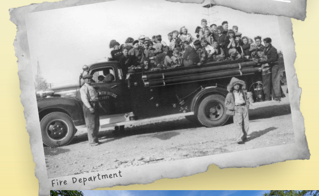
A road building crew - 1929
